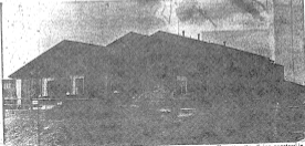
These new Seattle townhomes at Mission Viejo in a planned community for southeast Aurora offer attractive living quarters at as little as $24,900.
